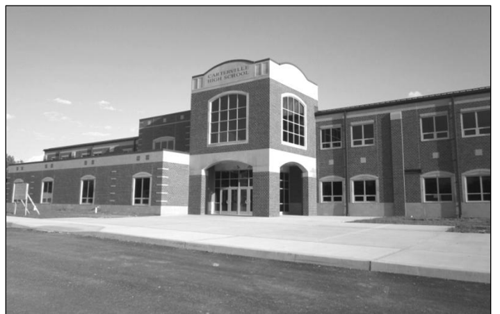
Looking virtually complete, this is a view of the front of the new high school on April 28, 2011.
